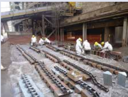
HLB bucket elevator chain
